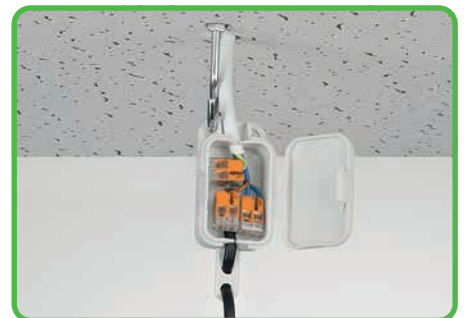
Pendant light connection in suspended ceilings
